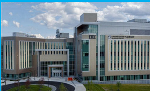
Emerging Technology and Entrepreneurial Center (ETEC) was awarded 2023 Green Building of the Year by U.S. Green Building Council of Upstate New York
