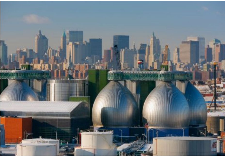
Wastewater Recovery Facility-Brooklyn
